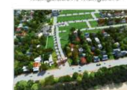
Emerald Bay Surathkal, Mangalore
